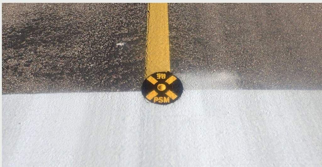
Photo 4 – Emergency RWY (TWY A) REPSM18R (New bolt in asphalt)
